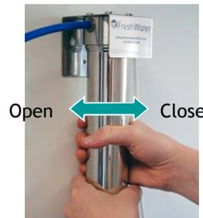
3. Leave the housing assembly on the bracket. Firmly grip the sump with both hands and turn to the left to release the seal. The sump of the filter will be full of water so position the bowl carefully to catch the residual water.
